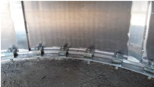
Silo Fixing Footings
