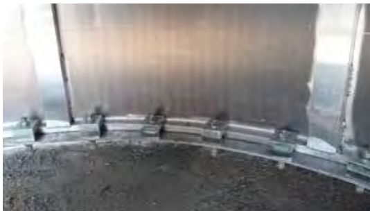
Silo Fixing Footings
